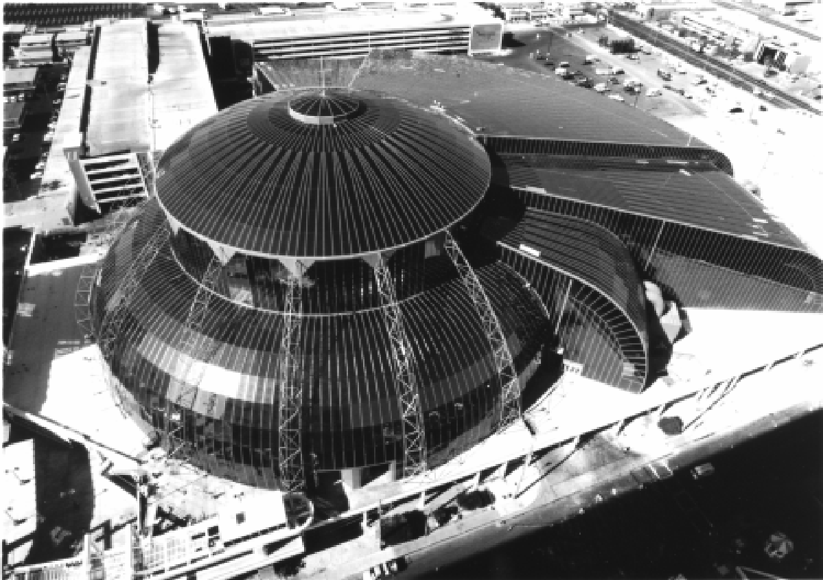
FIG. 5 Sloped SSG System
