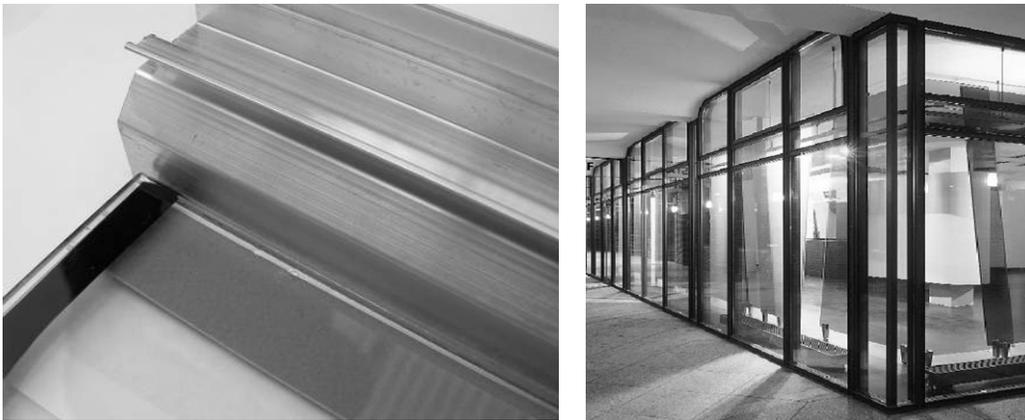
**Figure 1.** Bonding of laminated safety-glass panels to aluminum framework with pressure sensitive tape
